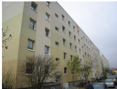
Figure 3. About 1995, this multi-storey building on the outskirts of Berlin was renovated and the exterior walls were supplemented with a rendered and ventilated cladding system.
