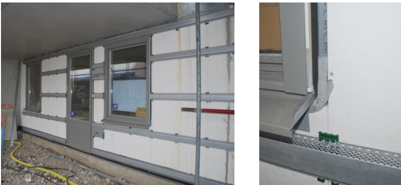
Figure 4. Arrangement of horizontal, vented metal supports with depth 25 mm (left) and a close up which shows the web perforation (right). The function of the green plastic spacers behind the supports is to level out unevenness in the substrate.
